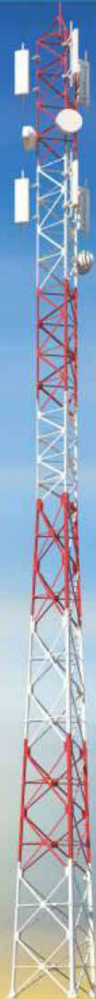
3 Legged Lattice Tower
